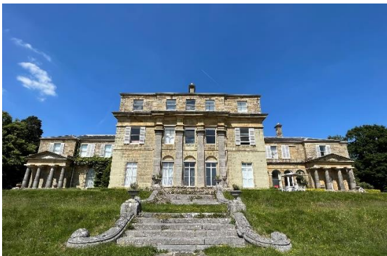
View looking north © T Messent
